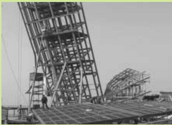
Construction of WSS floating set.
