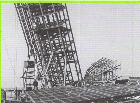
Construction of WSS floating set.
